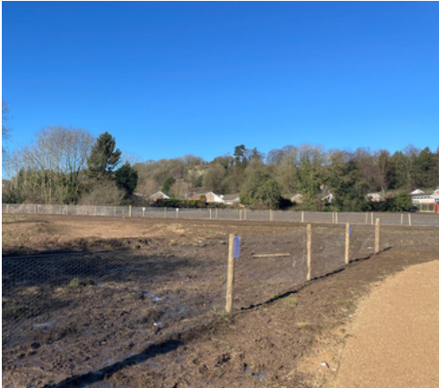
Fencing in place
