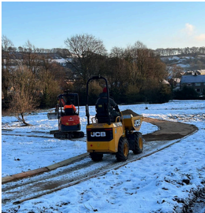
Work in the December snow
