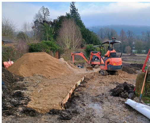
Working at the Yokecliffe entrance
